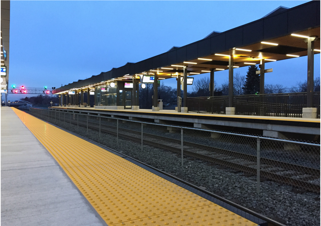
A platform edge at Weston Station installed with Armor Tile® Transit – Surface Applied.
