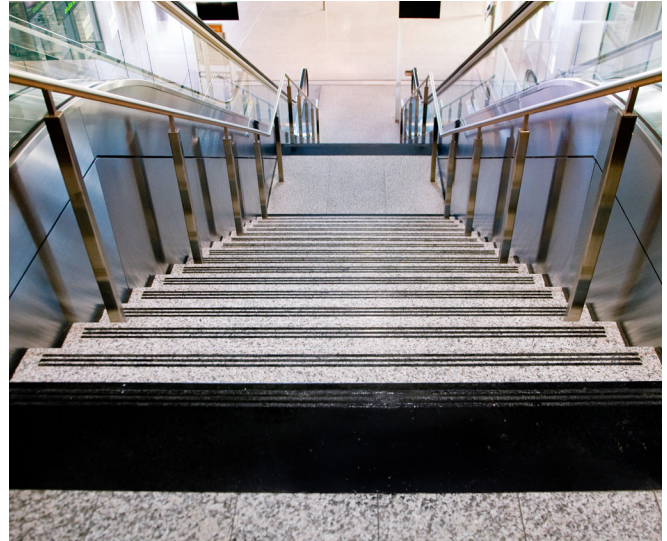
An example showing poor use of stair nosings. The light-coloured treads with black strips on the nosing create a marking pattern that is not perceived well by people with vision loss.
